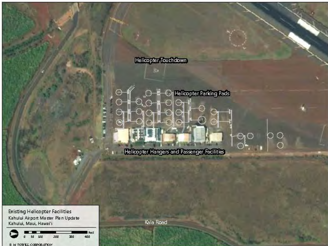
Figure 2-7 Existing Helicopter Facilities Terminal Complex
