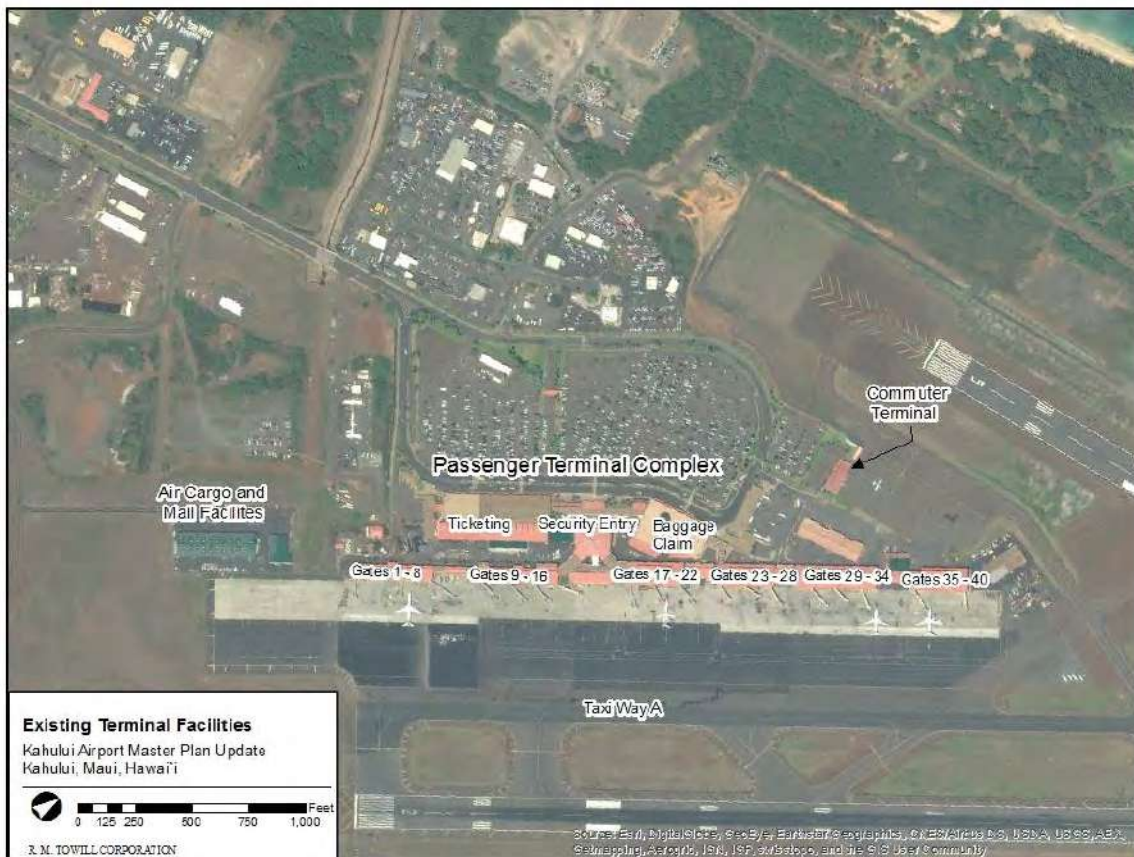
Figure 2-5 Existing Terminal Facilities
