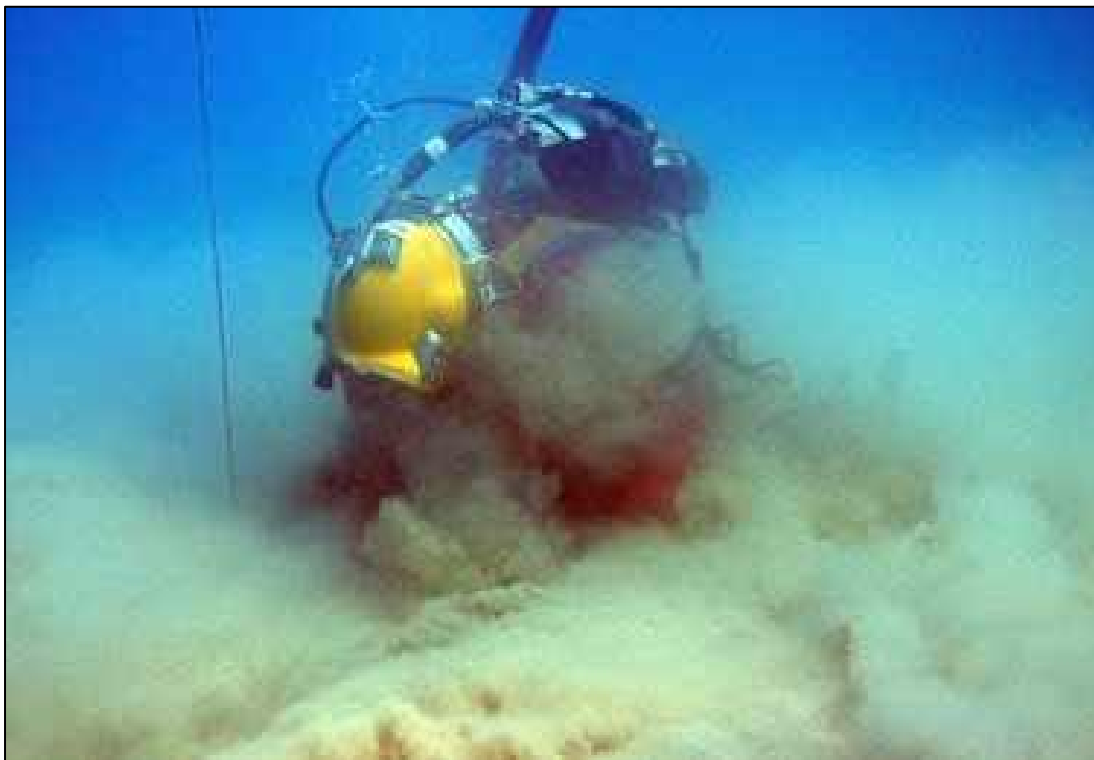
Figure 3-12 Surface supplied air (SSA) diver using a diver-operated dredge
