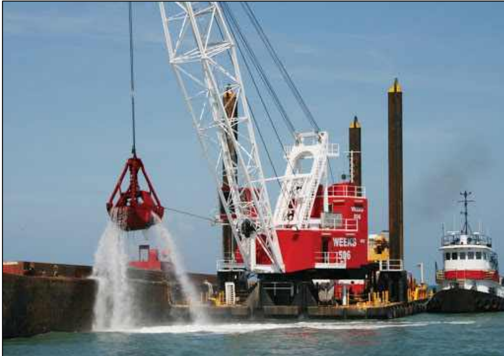
Figure 3-9 Example of clamshell dredging (IP Subsea)
