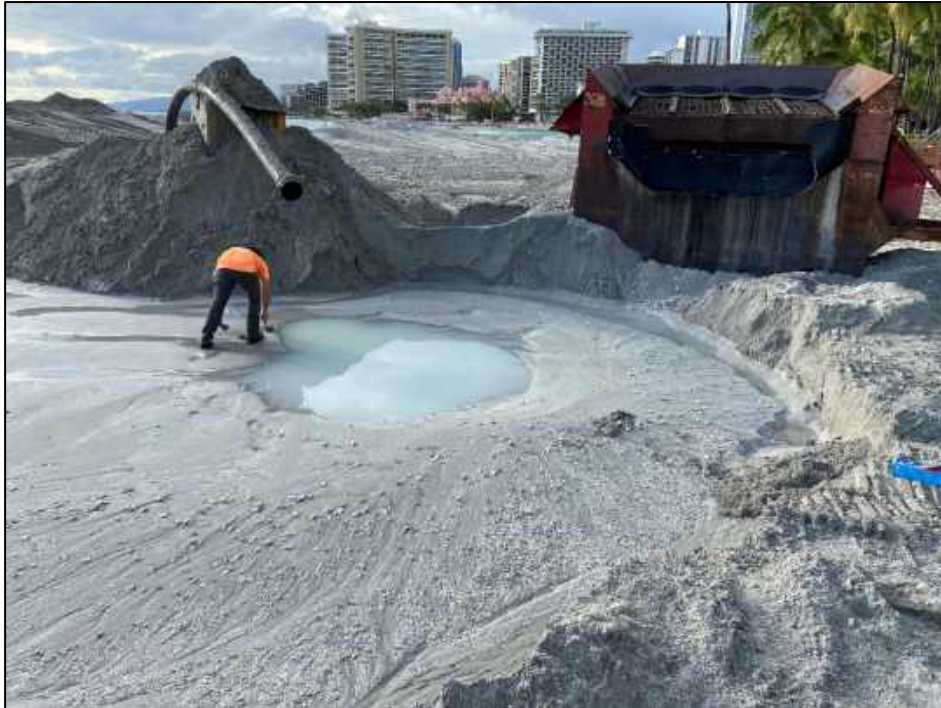
Figure 8-47 Screening process to remove cobble from offshore sand
