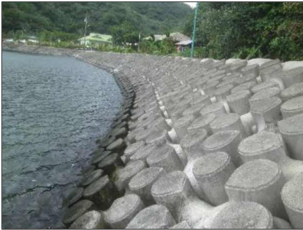
Figure 3-14 Tribar concrete armor units in American Samoa
