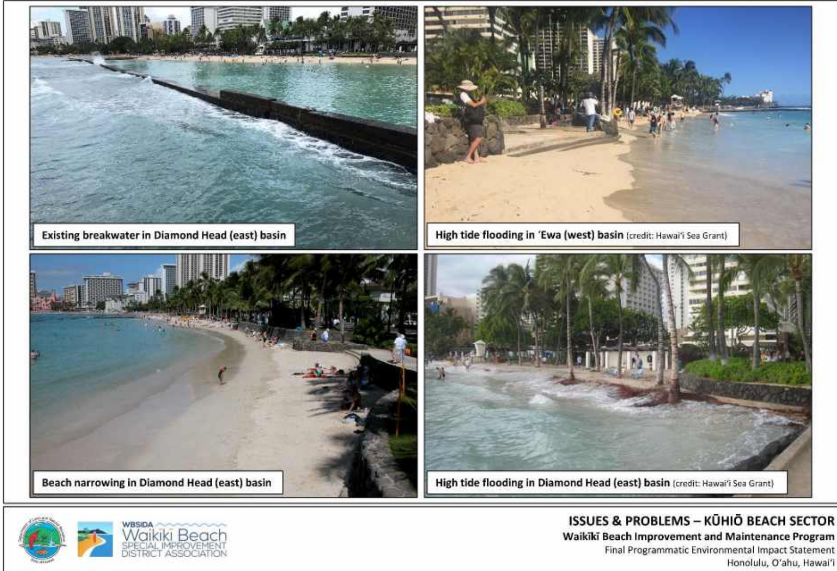
Figure 7-7 Issues and problems – Kūhiō beach sector
