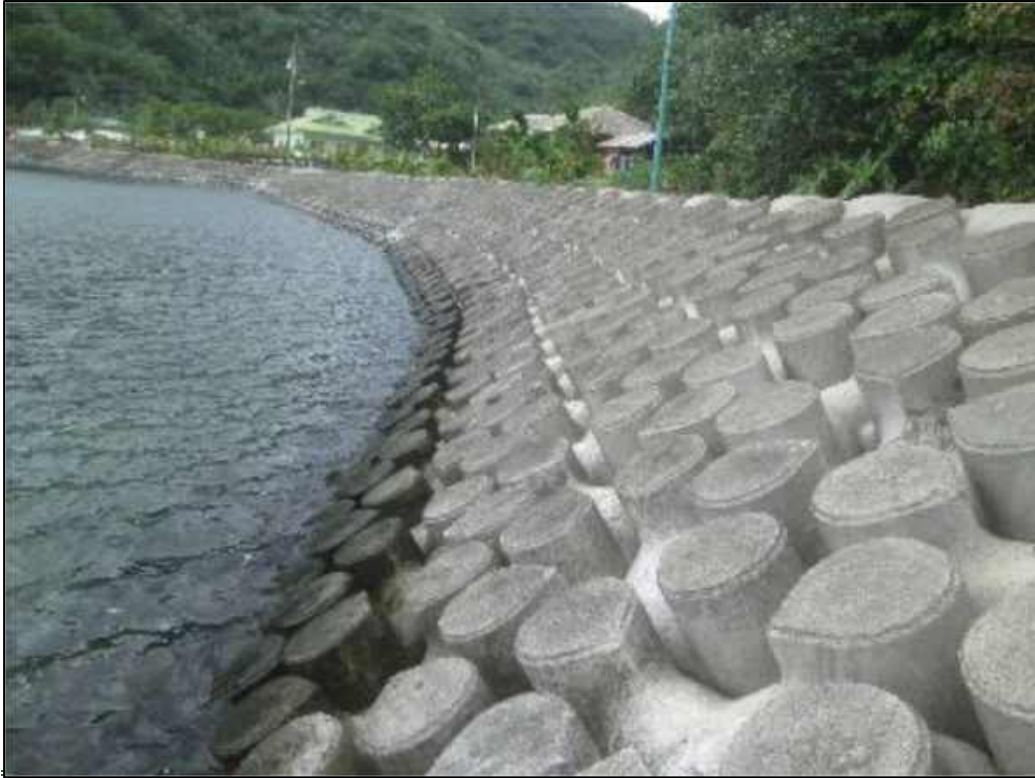
Figure 5-14 Tribar concrete armor units in American Samoa
