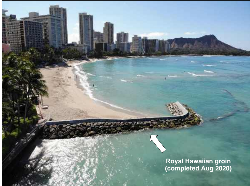
Figure 2-10 Conditions after reconstruction of Royal Hawaiian groin (August 2021)
