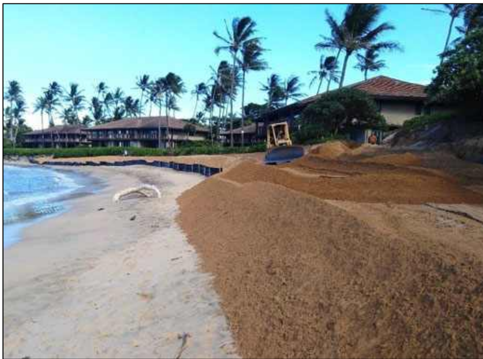
Figure 3-3 Small-scale beach restoration at Pā'ia, Maui (2016)
