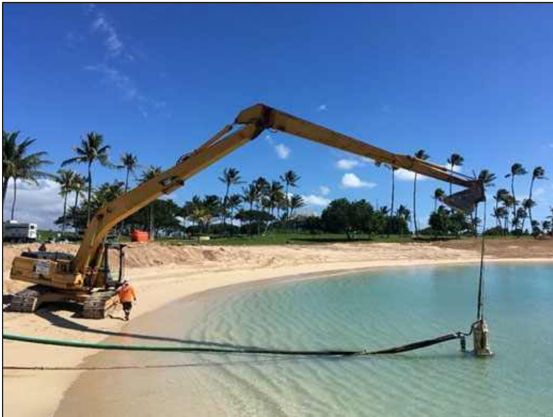
Figure 3-2 Sand pumping at Ko‘olina, O‘ahu (2017)
